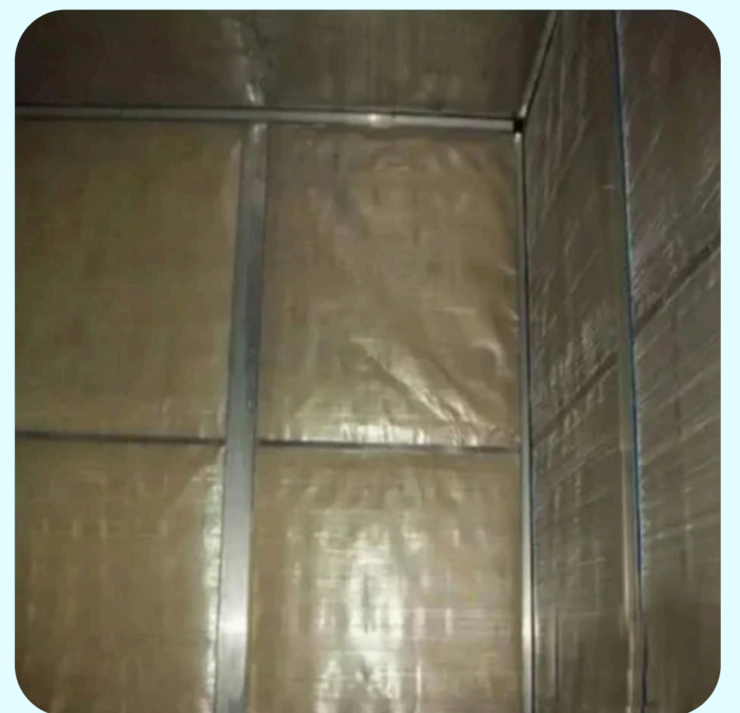
Room Acoustic Installation
