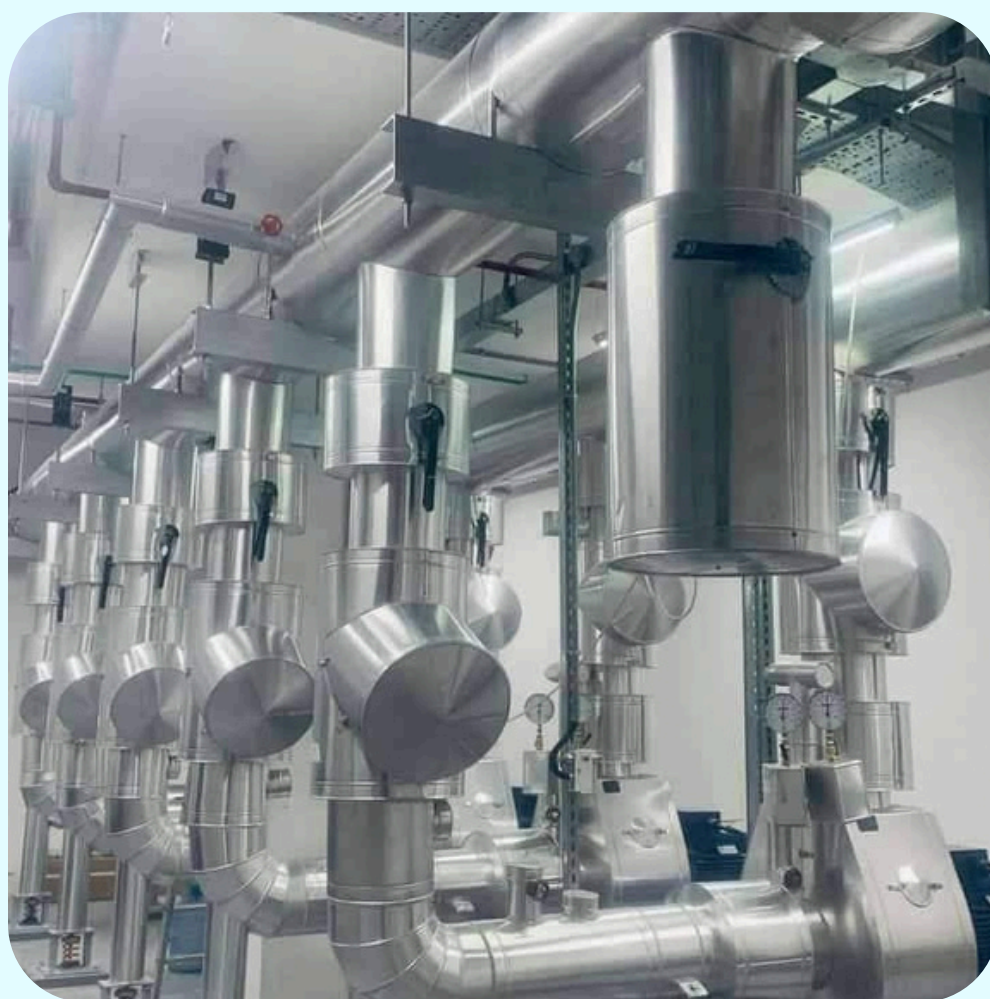
Cladding Installation
